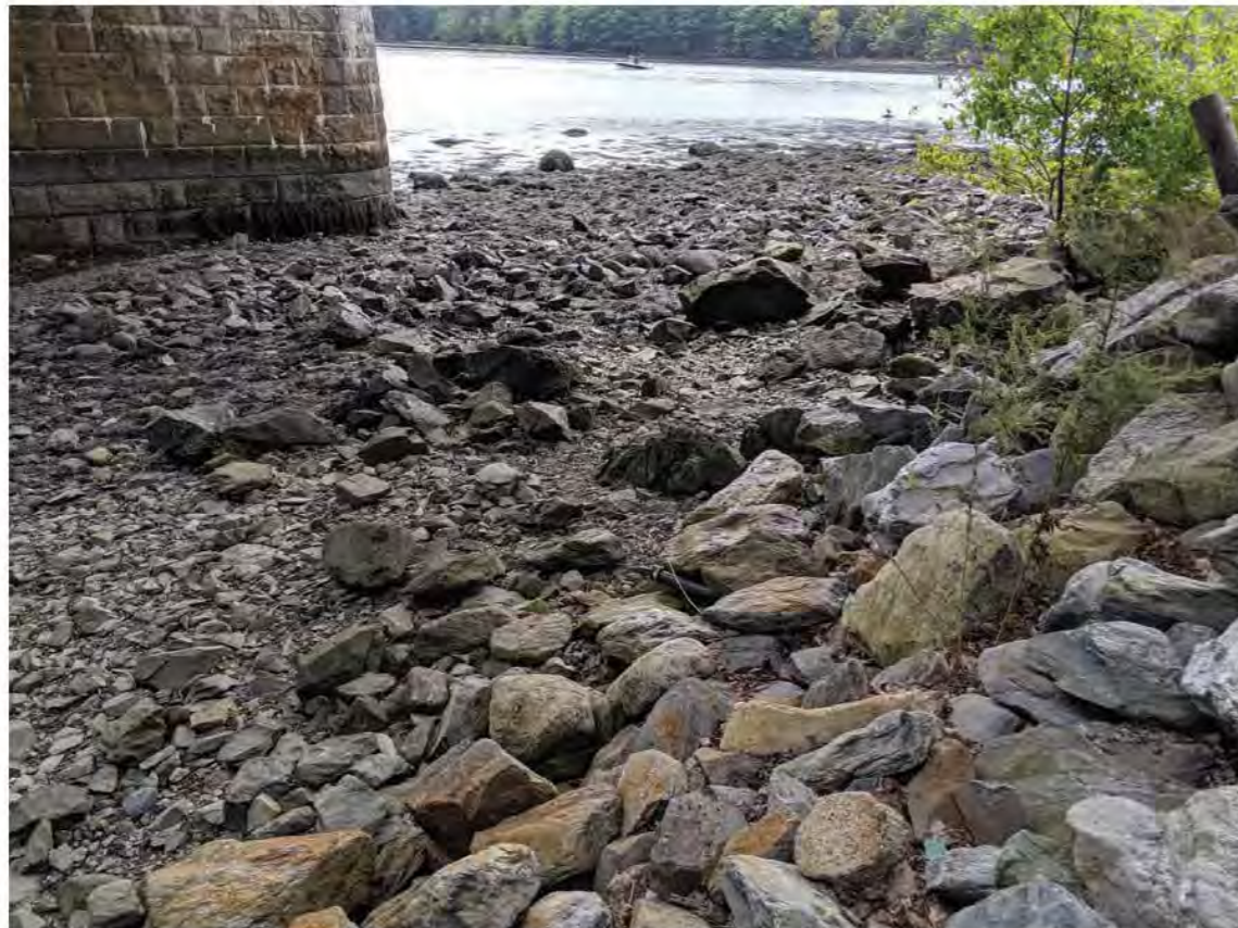
Existing abutment in Dover, facing west to show existing conditions.
