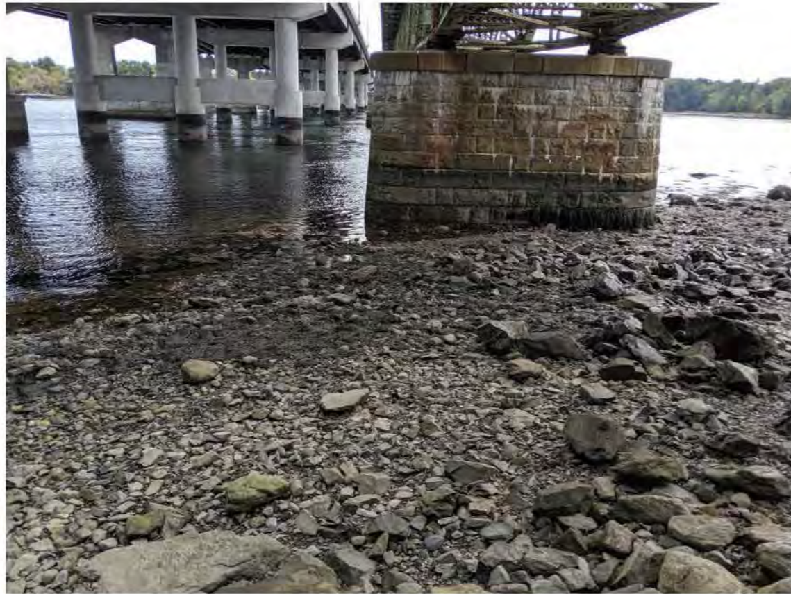
Existing bridge abutment, and proposed location of temporary stone fill causeway. (Dover, north side)
