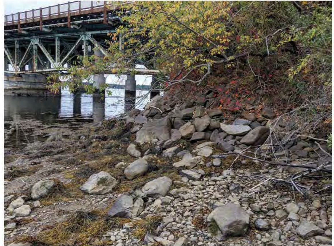
View toward existing abutment in Newington, and location of proposed temporary causeway.
